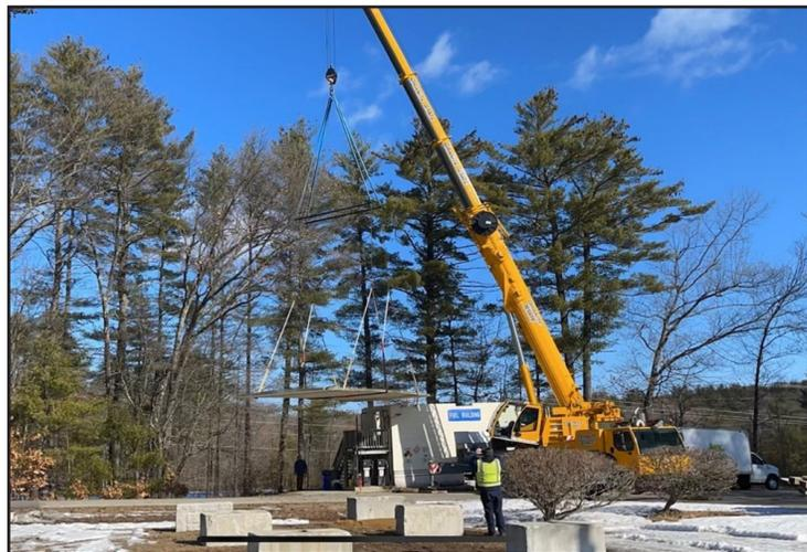
*Pictured Above: Fuel building concrete roof removal.*
